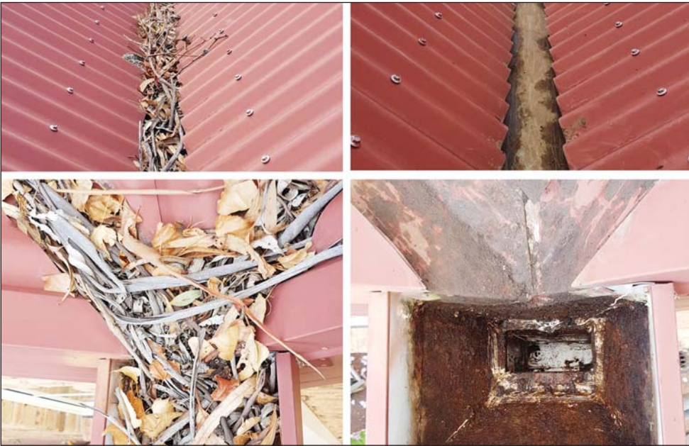
Debris in gutters act as kindling for embers (in the 'before' image on left). Gutter-Vac Tasmania professionally removed the debris (shown in 'after' image on right). (PS)
