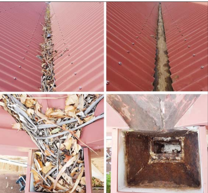
Debris in gutters act as kindling for embers in the 'before' image on left. Gutter-Vac Tasmania professionally removed the debris, shown in 'after' image on right. (PS)
