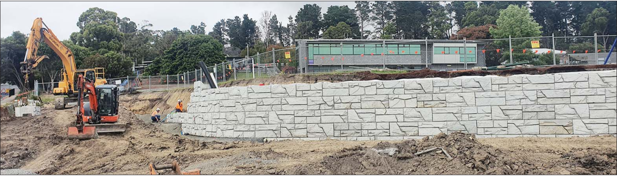
Construction is underway on a new carpark and bus lane at Calvin Primary School in Kingston. A retaining wall is being built to level off the play area, while providing further parking spaces below. Construction is expected to continue for the next few months. (PS)
