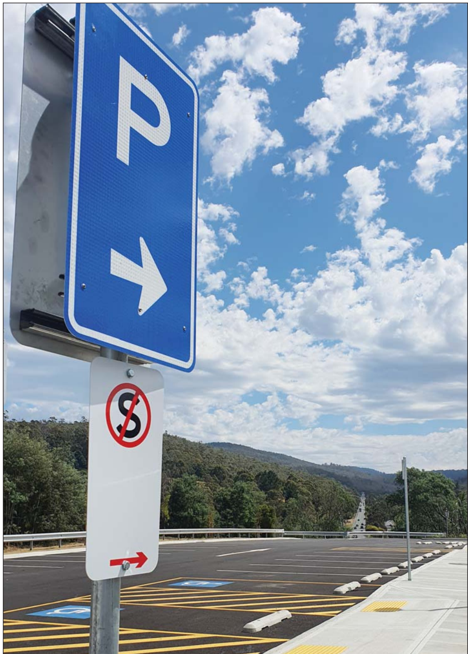
The Park and Ride parking at Browns Road is nearing completion. The parking area and roads are sealed with kerb and footpaths. Landscaping with shrubs and trees is also complete. (PS)
