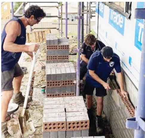
Nathan and his team laying a brick veneer wall for a new build recently. (PS)
