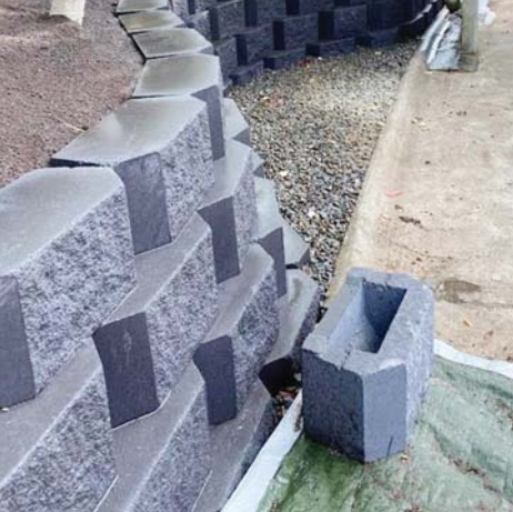
Knights of the Trowel Bricklaying specialises in dry stack retaining walls. (PS)
