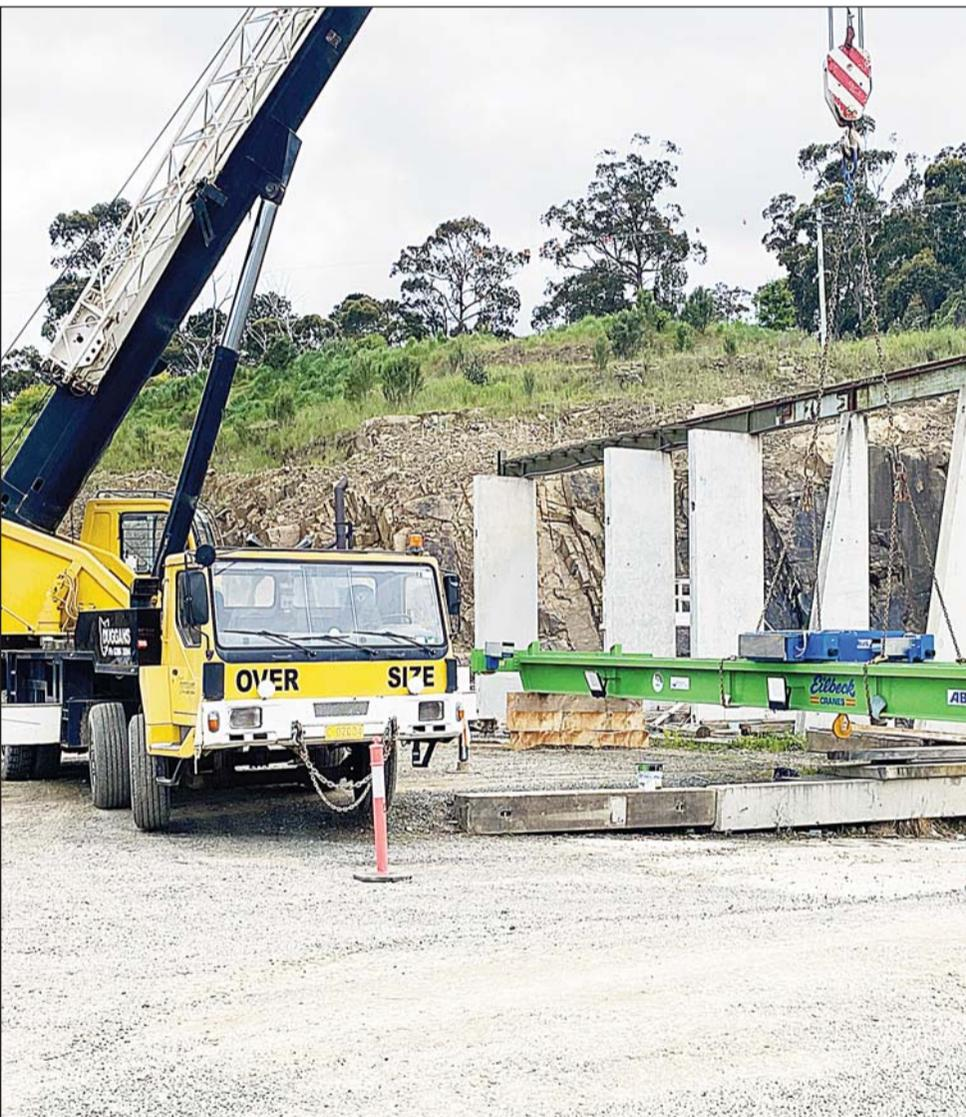
An additional 20-tonne gantry crane joined the team at Duggans Precast Factory in late 2021 to improve capacity and efficiency. (PS)
