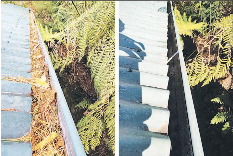
Pine needles gathered in a roof gutter for four months are removed during professional cleaning by Gutter-Vac Southern Tasmania. (PS)
