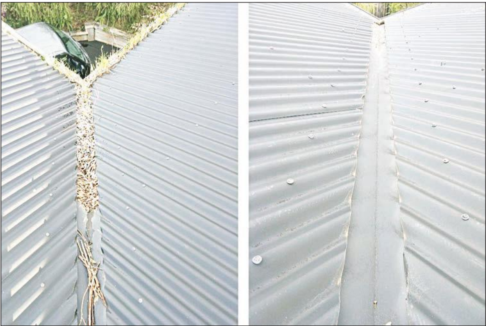
Debris in gutters acts as kindling for embers. Gutter-Vac Southern Tasmania professionally remove the debris. (PS)
